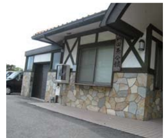
"Yamadahara Kaikan" (Community Center) is in front of you. Beside the front door of "Yamadahara Kaikan" a public phone is placed. Use it call a taxi.
